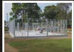
Erecting the framing
