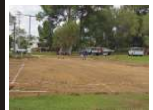
Marking out the site
