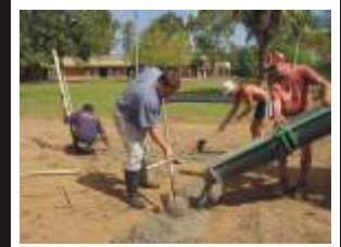
Preparing the footings
