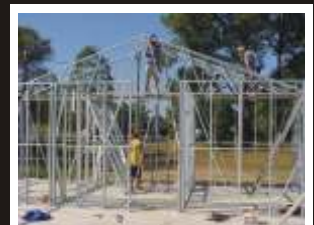
Attaching the roof trusses
